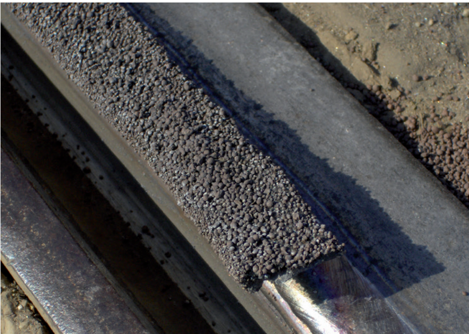
Excellent weld bead appearance, also in rail crossings and bends
